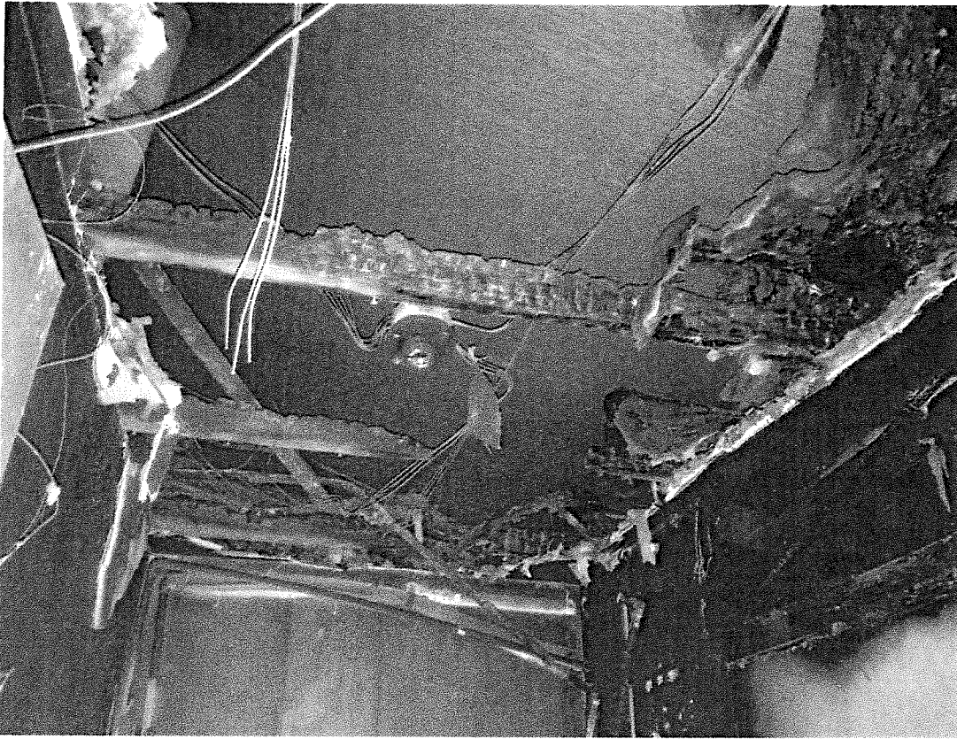
Photo 3 – View of Damaged Destroyed Roof Trusses Over Utility Room
